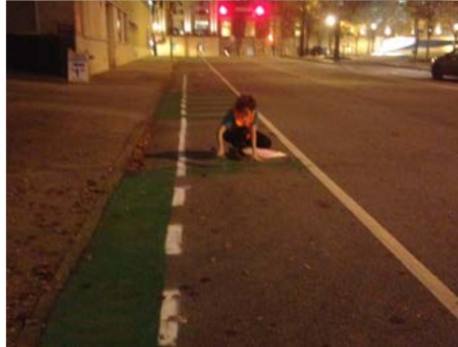
5 feet was measured from the outer bike lane striping and the bike lane was re-striped. The remaining 3 feet was filled with bricks to level with the curb and paint. Intersections were painted green and the bike lane was striped green.
